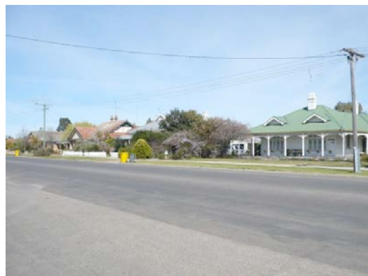
Scott Street in Warracknabeal contains many fine houses that demonstrate the growth and prosperity of the town during the early 1900s, interwar and early post-war periods.
