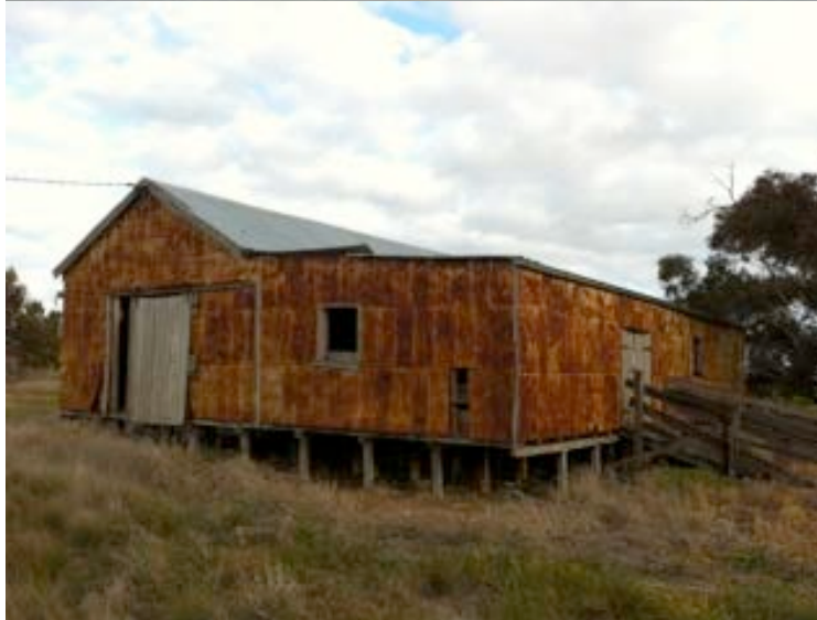
Figure 5: Kerosene Tin Shearing Shed, Woomelang
